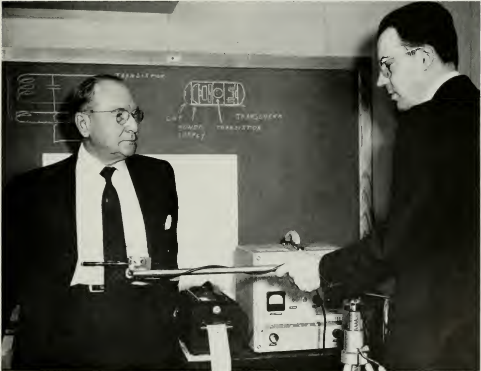
Dr. John T. Farrar (right) holds antenna against Dr. V. K. Zworykin to demonstrate how FM radio waves are picked up from "radio pill" as the capsule passes through the body.
